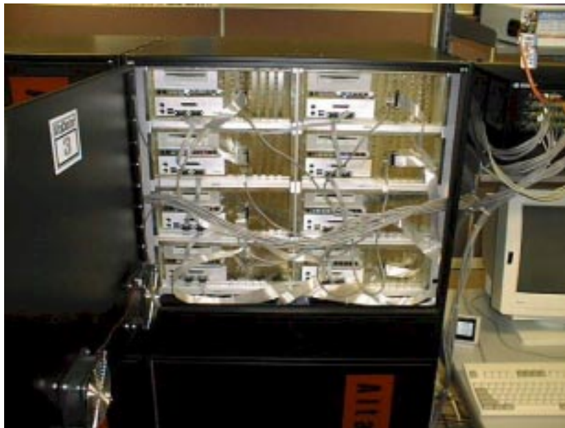
Figure 2: A Peek Inside the Roadrunner.
