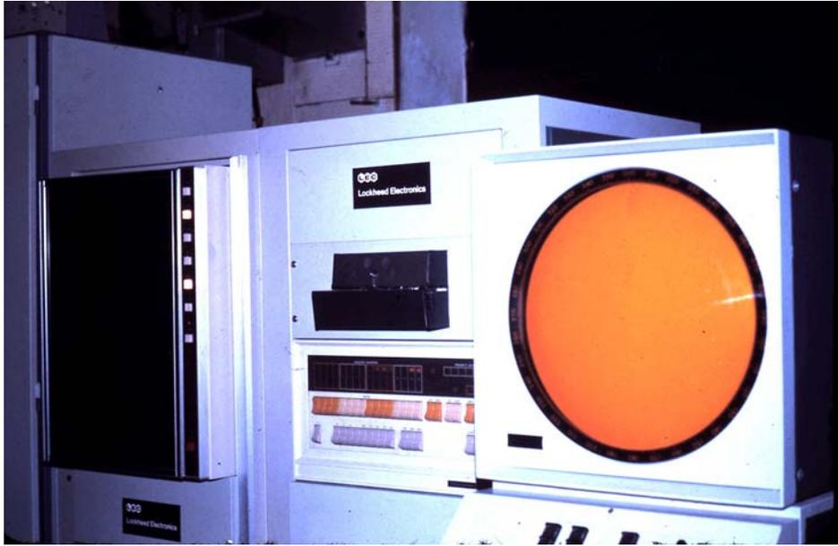
Figure 1 – MAC-16 demonstrating Air Traffic Control in Italy
