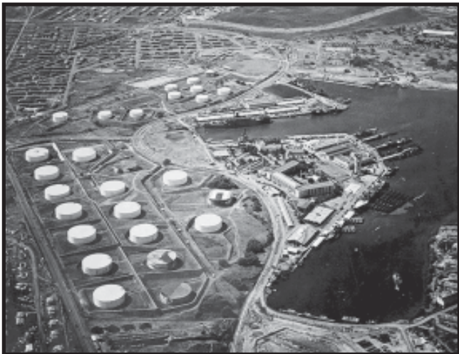
Figure 2. Submarine Base, Pearl Harbor and Adjacent Fuel Tank Farms, 13 October 1941. This is a view of the upper oil tank farm located on the east side of the Pearl Harbor naval base. The lower tank farm was located between Hickam Field and the naval base (see Figure 1 for oil tanks in the lower farm). Note the attempts at camouflage. Two of the tanks in the foreground are painted to resemble terrain features. The third, closest to the submarine base, is painted to resemble a building. 87
